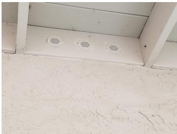
Ember-resistant vents for installation in an Olivenhain home
